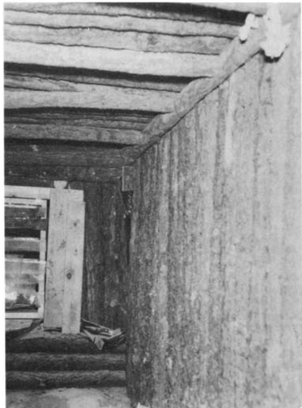
Fig. D.2. Undamaged interior of a Small-Pole Shelter after blast testing at the 53-psi overpressure range. Large buildings would have been completely demolished.
