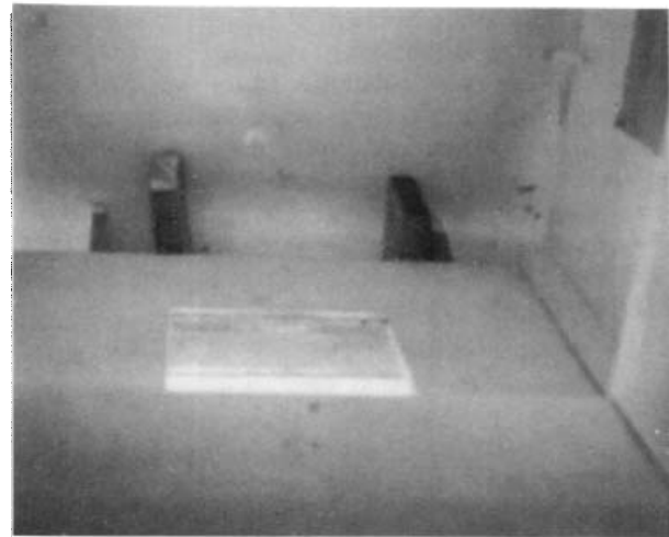
Fig. F.4. View from Below the Exit, Looking Up the Multi-Purpose Emergency Exit Housing. The top is shown supported in a tilted position by two 6-inch-wide boards placed between a wall and the top.
