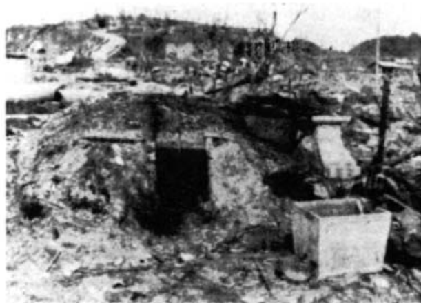
Fig. 1.5. Undamaged earth-covered family shelter in Nagasaki.
